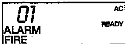
Typical Fire Emergency Display
